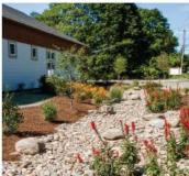
Bioretention - Dry Condition Attractive in both wet and dry conditions.
